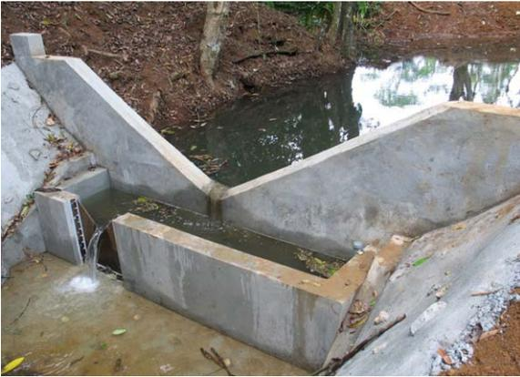
**Figure 3.** Two-stage weir structure at PAS catchment outlet. The top width of the concrete 120° V-notch weir is 4.4 m. Photo by F. Ogden.
